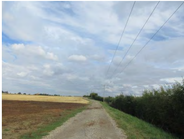
Photograph 17. Farm access track towards substation and transformer location. Load approaches camera. Negotiable with caution and confirmation of overhead clearances to power lines. Road width 3.4m.
