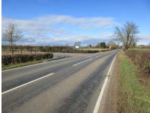
Photograph 1. Access to farm from Sturton Road at OS Ref SK 89173 77603. Load moves away from camera and turns left. Negotiable.
