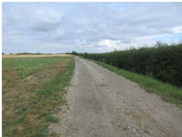
Photograph 18. Farm access track towards substation and transformer location. Load approaches camera. Negotiable with caution and confirmation of overhead clearances to power lines. Road width 3.4m.
