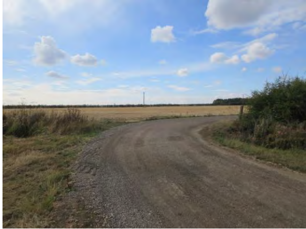
Photograph 4 First right hand bend on farm track. Load moves away from camera. Negotiable. Temporary road widening via plates or hardcore could be undertaken if required to widen road surface but this is not expected to be necessary.
