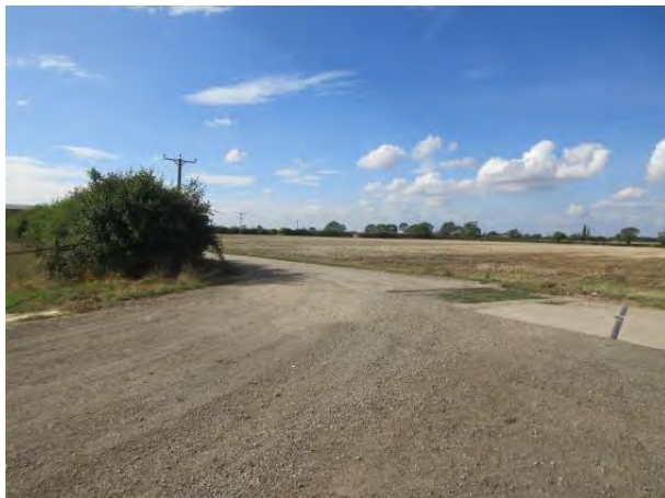
Photograph 6 First left turn on farm track. Load moves away from camera. Negotiable. Temporary road widening via plates or hardcore could be undertaken if required to widen road surface but this is not expected to be necessary..
