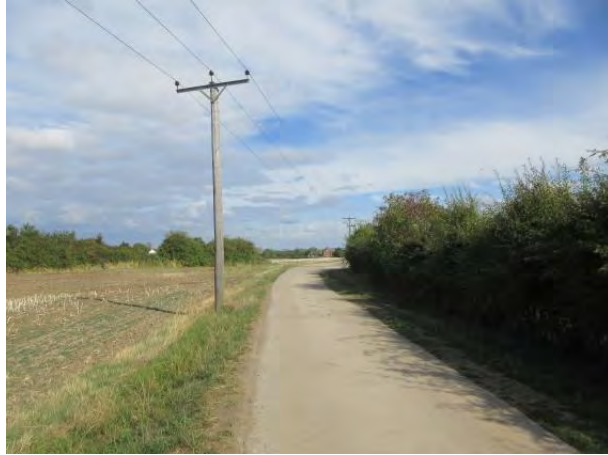
Photograph 7. Farm access track towards stables. Load approaches camera. 6m distance between power line pole and hedge. Road surface measured as 2.8m on this section. Temporary road widening via plates or hardcore required to widen road surface. As on private road confirmation of overhead clearances for electricity wires necessary.
